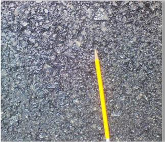
BinderTekk polymer modified asphalts are the newest generation of binder technology that can be engineered to address the specific level of strain tolerance needed for a particular job. BinderTekk is the solution for providing rut resistant base, intermediate, and surface HMA mixtures that are much more crack resistant than conventional HMA layers, whether placed as single or multiple lift pavement designs.
